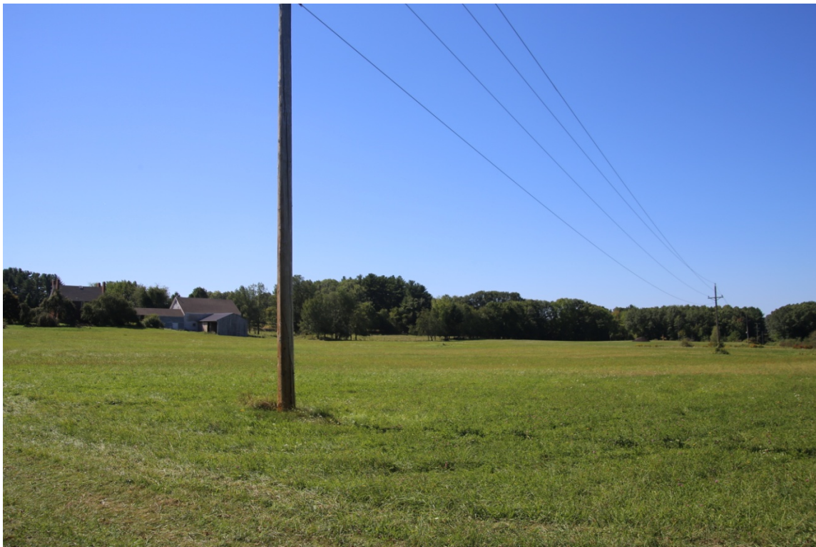
Newington Center Historic District - Frink Farm, facing southwest from Nimble Hill Road at Project location, showing existing distribution line to be removed.
